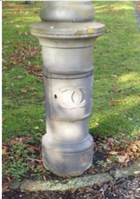
Example of base of streetlamps in the Chetwynd Barracks site.
