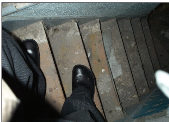
Stairs showing broken step
