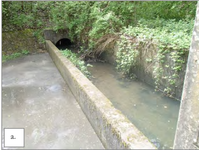
a) Concrete culvert channelling Daisy Farm Brook beneath the A610. b) Overflow ditch which runs along the southern boundary.
