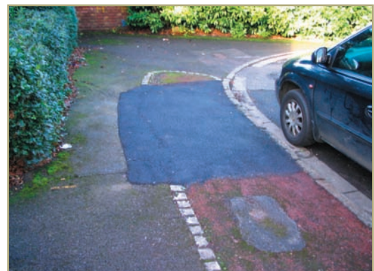
Erosion: loss of stone setts
