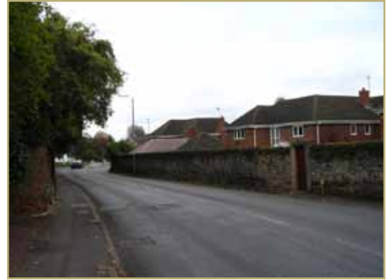
Stone wall of former nursery
