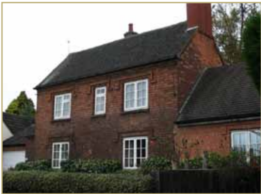
Cottage with brick drip-moulds
