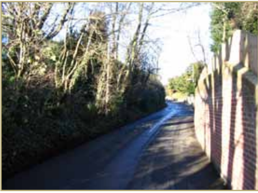
'Sunken' nature of west end of Hallams Lane
