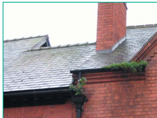
Blocked guttering on 52-56 Nottingham Road
