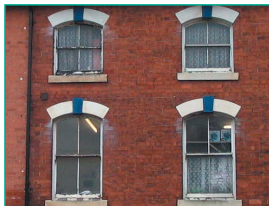
Peeling paint on original sash windows, number 72
