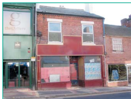
Oversized display fascia has replaced original cornice
