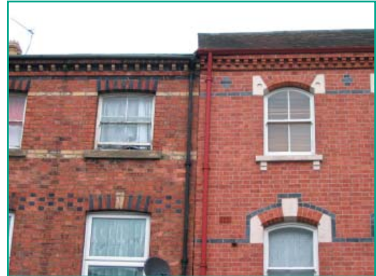
Dentilated eaves, polychrome brickwork
