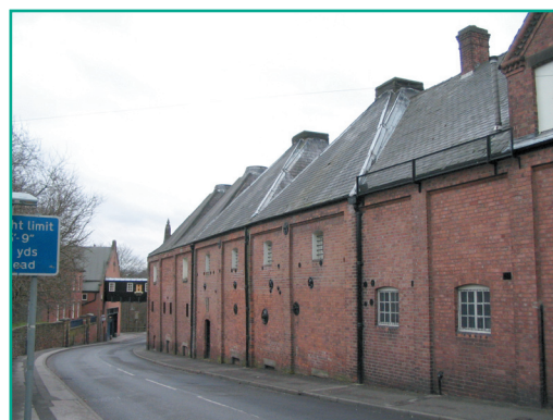
Pilasters/blind arcading and malt kiln roof structure
