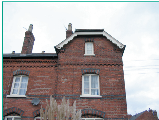
Half-hipped roof structure
