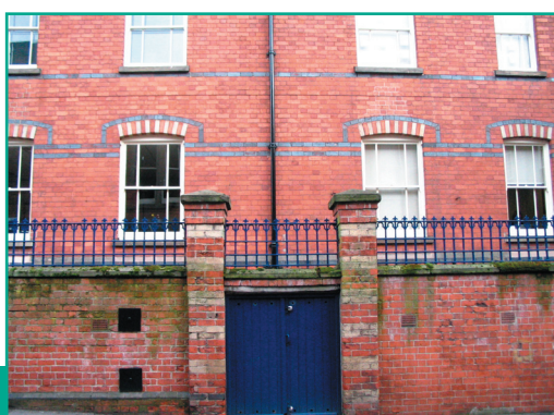
Cast iron railings, blue brick and buff brick banding
