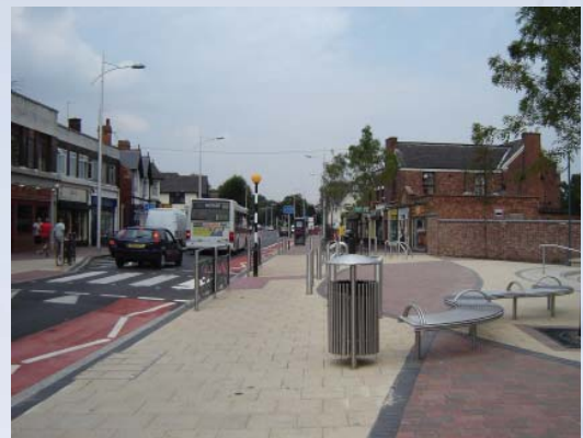
► Improvements to High Road at Broadgate Park
