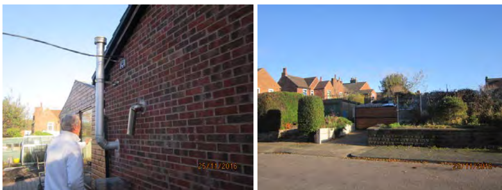
Outbuilding and attached log cabin Vehicular access
