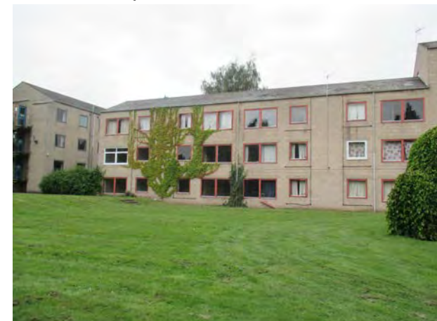
Image 6: Existing college residential accommodation
