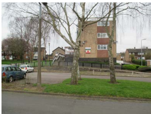
View from Melbourne Road
