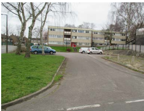
Car park and access
