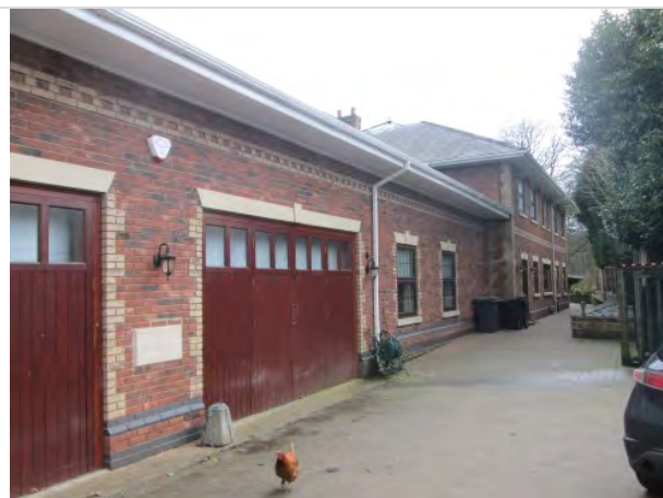
↑View of the northern façade of Temple Lake House which faces No.7B Edward Road
