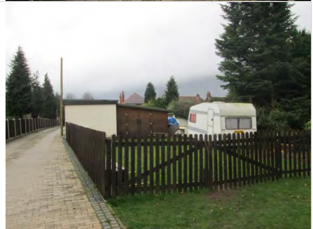
↑Existing outbuildings to the east of the private access which lie within No.53's garden would be demolished
