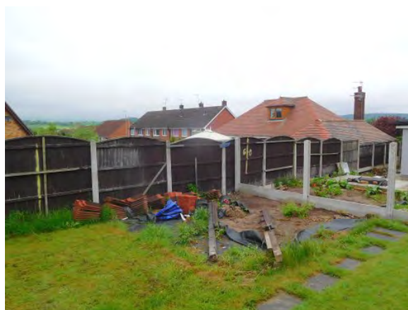
View from site looking towards no. 53
