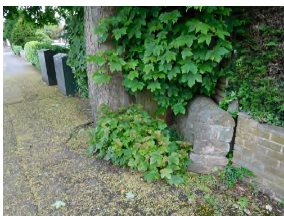
Damage caused by tree to the wall and footpath.
