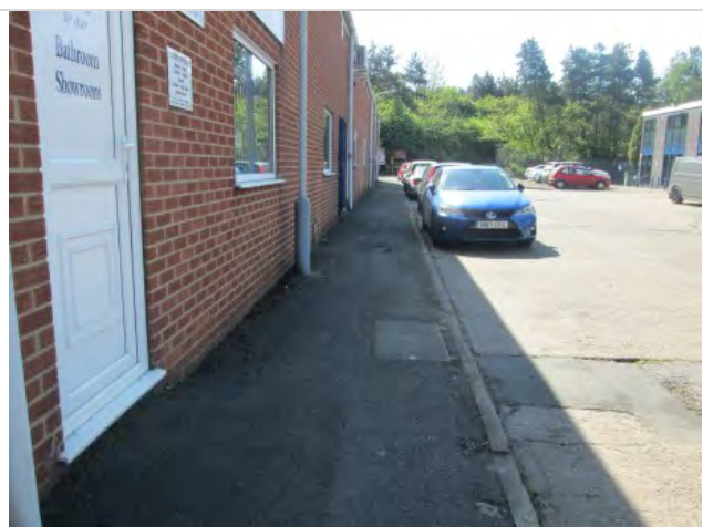
↑Pavements either side of the central section of Soloman Road provide links to Coronation Road where there is a nearby bus stop
