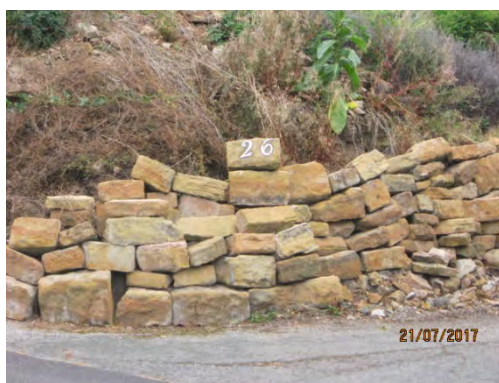
Collapsed section of the wall
