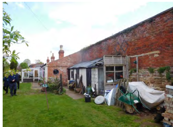
Existing outbuildings to south west of property.
