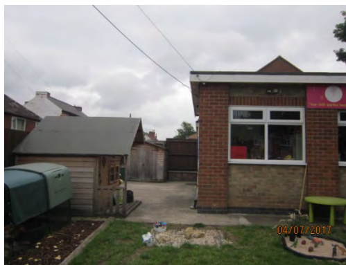
Northern side of building
