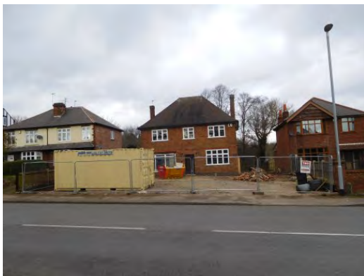
Previous view of property hedge removed and site cleared
