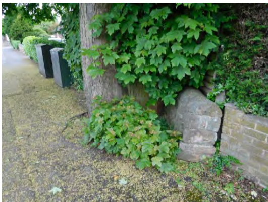
Damage caused by tree to the wall and footpath.
