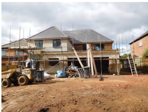
Recent rear view of property.
