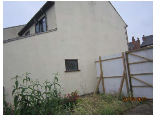
Side elevation of 125 Brookhill Street
