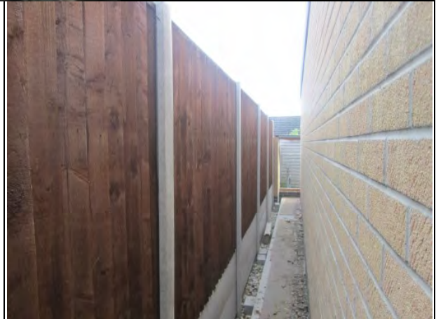
↑ View of the gap to the north boundary. New fence boundary treatment has also been erected by the applicant.
