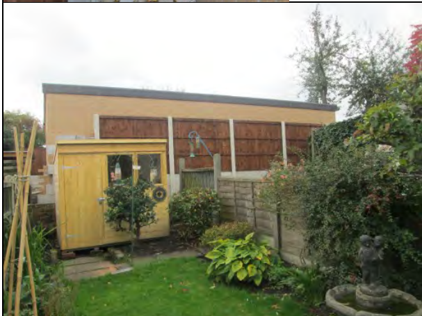
↑ View of the rear wall of the outbuilding from neighbouring No.78 Greenhills Road's garden to the north
