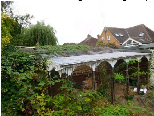
Oblique view of rear, showing no. 44 (to the west) in the background.
