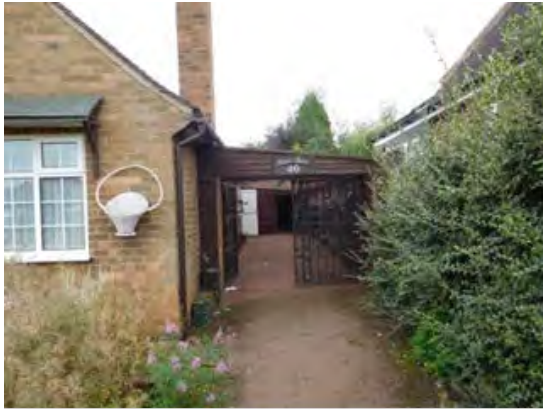
Side view of frontage, showing car port.
