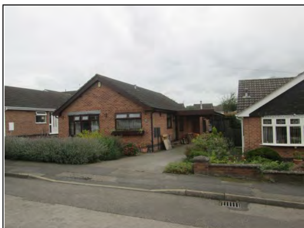
↑ View of the application site. The kennel outbuilding is not visible from street view.
