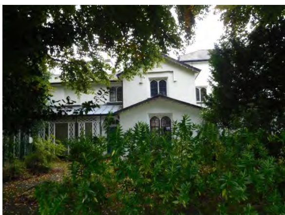
Dagfa House, viewed from Salthouse Lane
