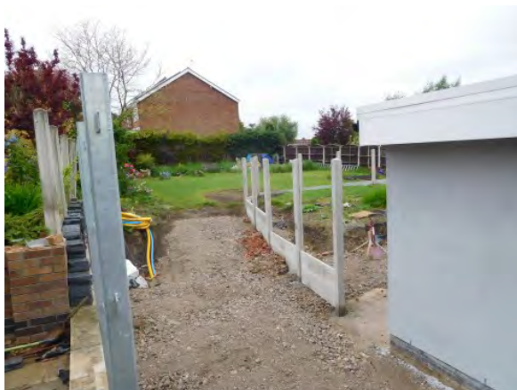
View from the access towards no. 11 Kirby Close
