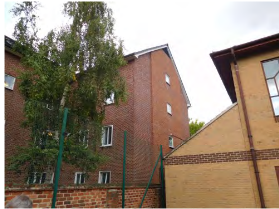
Relationship of former sports hall to adjoining student block.
