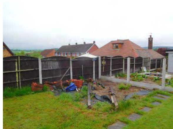
View from site looking towards no. 53 Mill Road.
