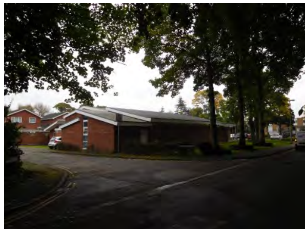
View of the Free Church and The Cloisters.
