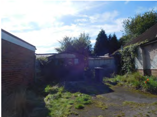
Garage and outbuildings on the left.
