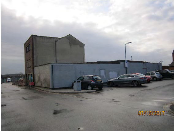
Chilwell Road frontage and Wilmot Lane public car park
