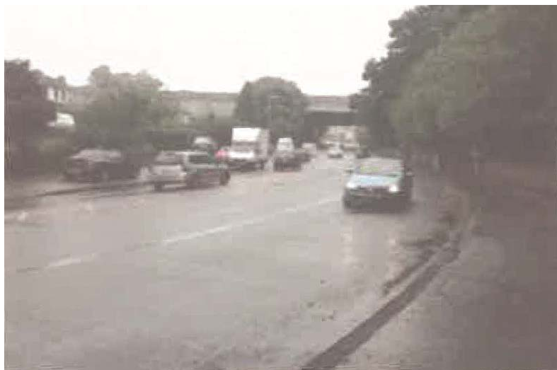
Illustration 15: M1 Motorway Bridge
