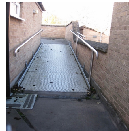
Regency Court: multi-level with many steps around scheme, slippery metal ramp to enable access for one person
