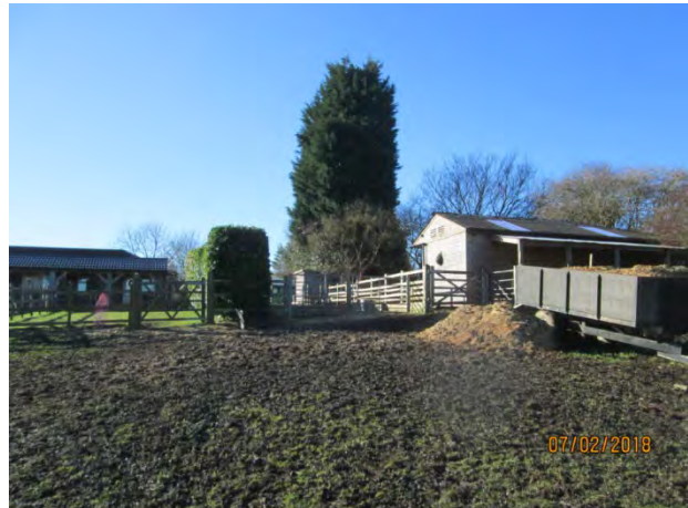
Stable block to south west of application site. Stable block is owned by applicants.
