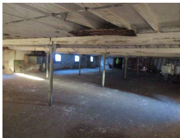
Malting interior; low ceilings & columns
