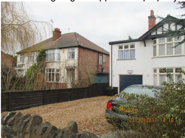
Looking south east towards front of no. 417 and application property (left) and no. 421 (right).
