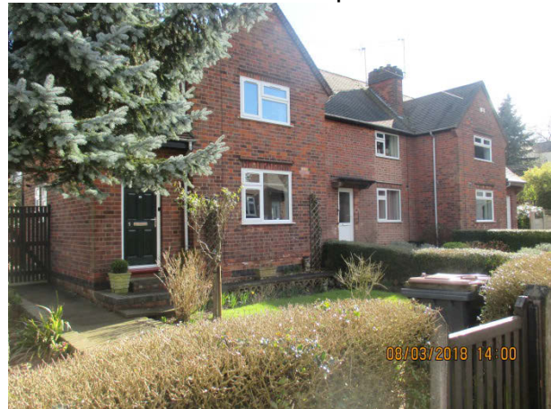
Front of no. 1 Henson Square (left).
