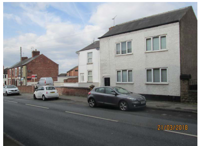
View of No. 73 and bin store from the south side of Main Street.
