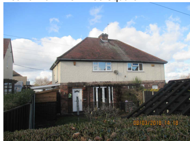
Rear of no. 3 Ash Tree Square.
