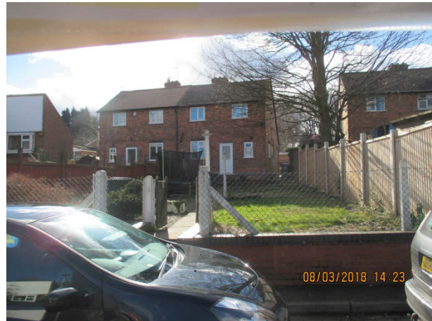
Rear of no. 7 Ash Tree Square
