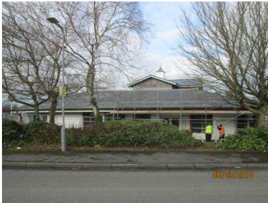
View from the north from Mornington Crescent.
