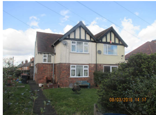
Rear of no. 1 Ash Tree Square.
