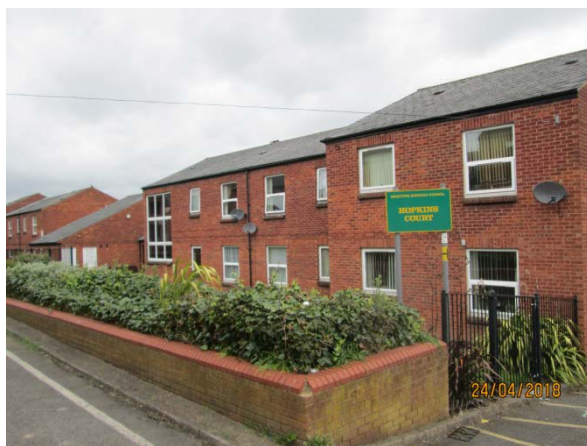
Central Block taken from east boundary.
