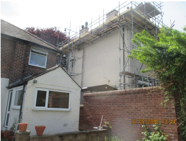
Looking west towards no. 3.
