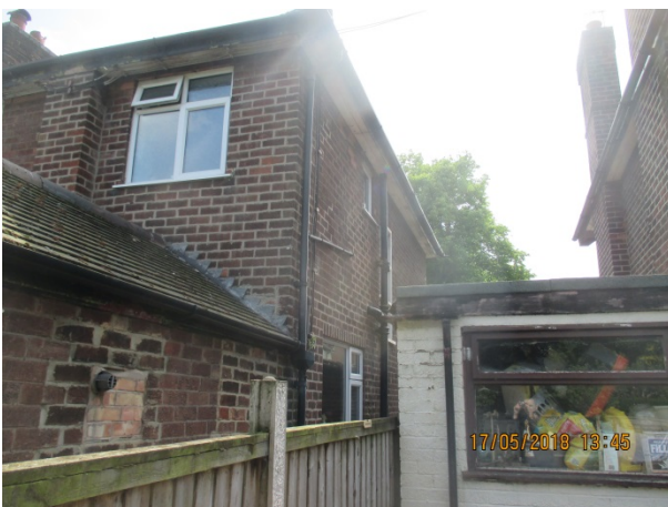
Looking south west towards boundary with no. 7.
