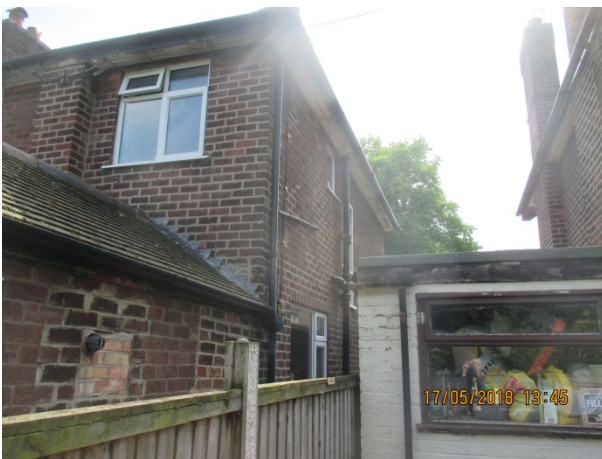
Looking south west towards boundary with no. 7.
