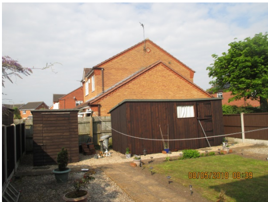
View from rear garden of no. 105 Haddon Crescent
