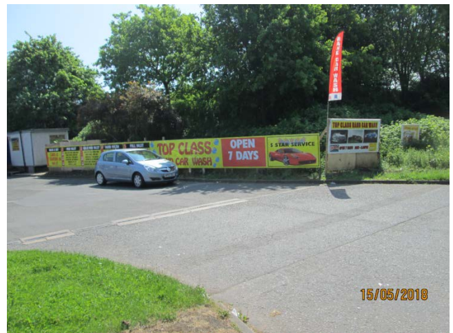
Signs to be altered and any remaining hoarding to be removed, in accordance with application 18/00261/ADV.
