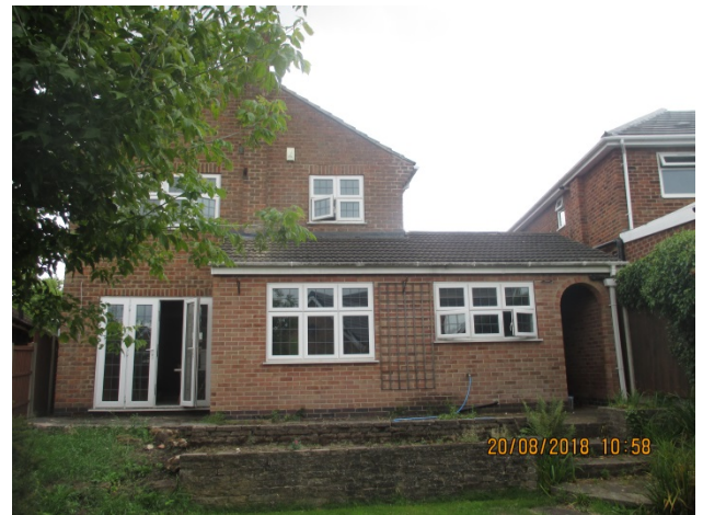
View of north west (rear) elevation
