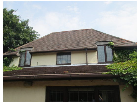
Existing rear roof view.
