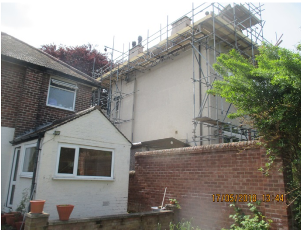
Looking west towards no. 3.
