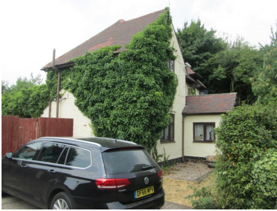
Front/Side Elevation from driveway.
