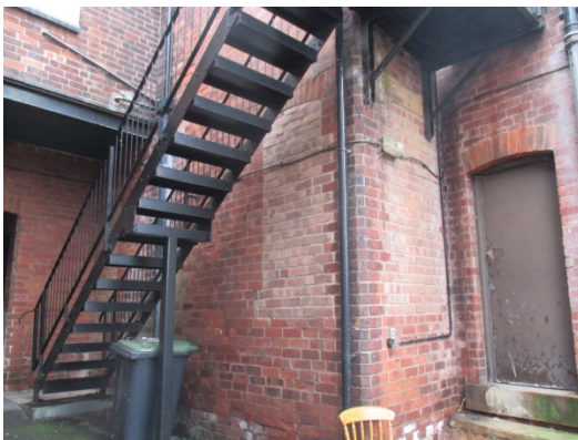
Rear of 250, former window openings
