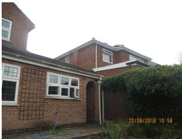
View of rear/side boundary with no. 4
