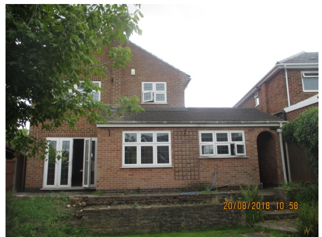
View of north west (rear) elevation
