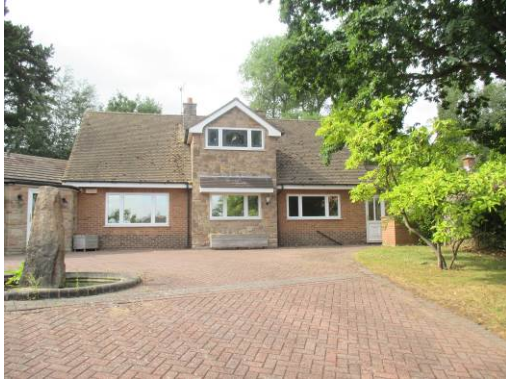
Extension prior to demolition
