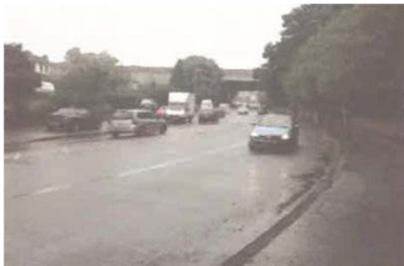
Illustration 15: M1 Motorway Bridge
