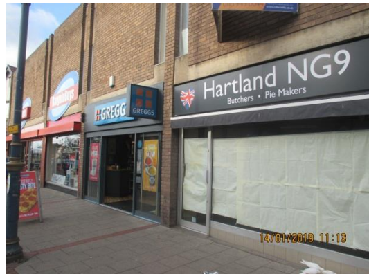
Looking west towards no. 46 (Bargain Buys), no. 44 (Greggs) and application site.
