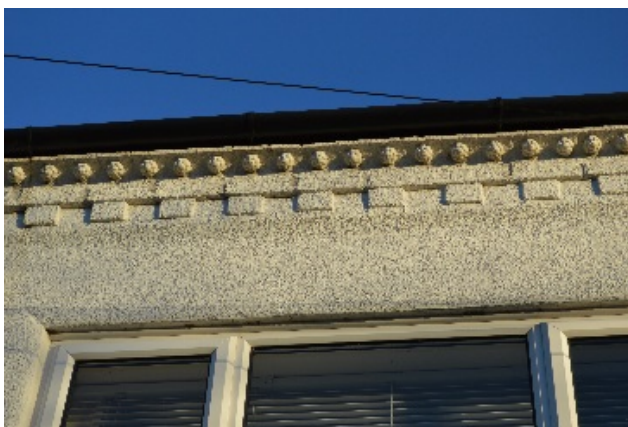
Inappropriate brick rendering masks original brick detailing
