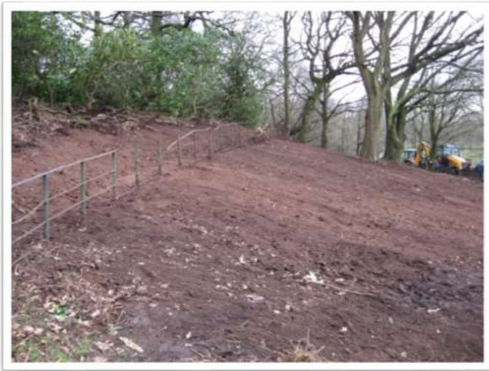
Earth movement and full rhododendron clearance reveals line of “estate” fence.
