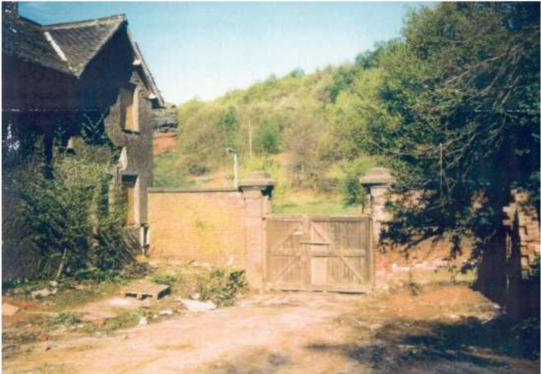
Figure 15 – Gardener's Cottage Pre-demolition
