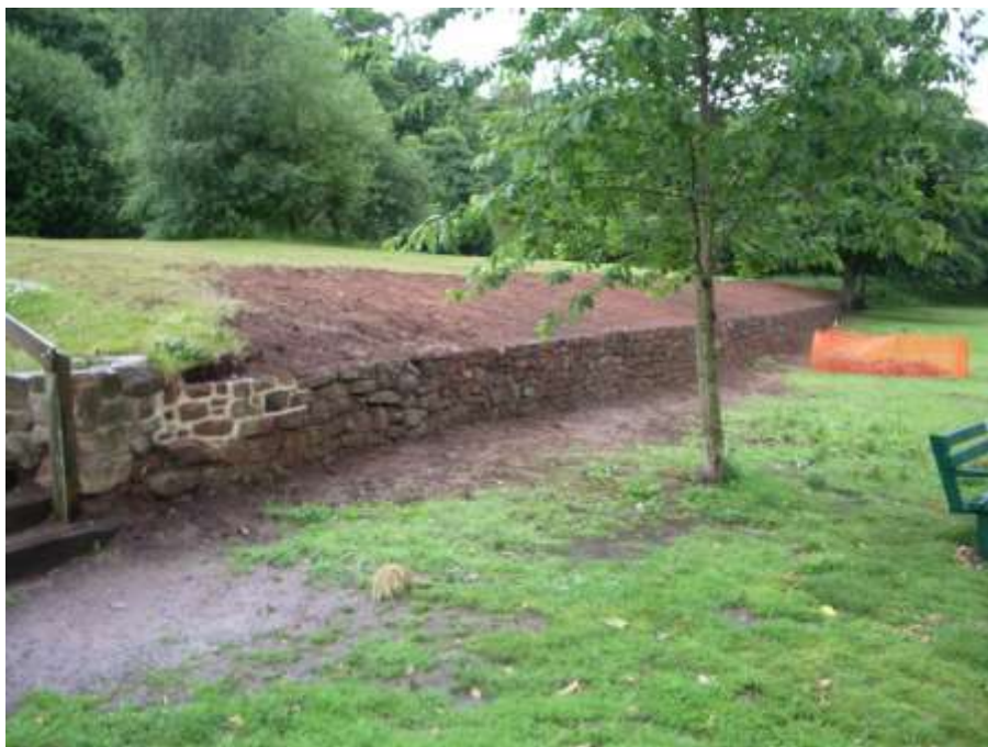
Figure 38 – Bramcote Hills House Wall After
