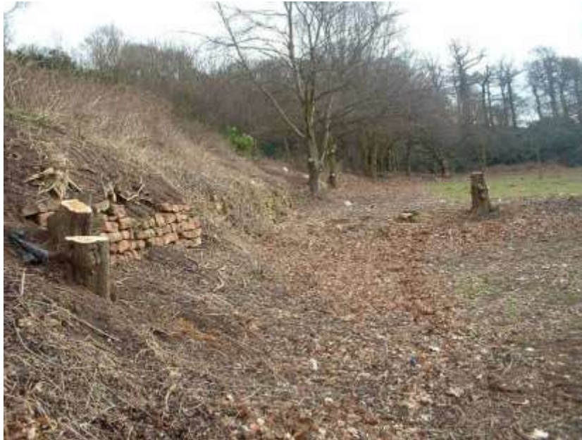
Figure 37 – Bramcote Hills House Wall Before
