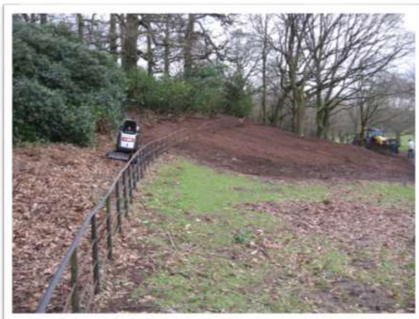
Link between previous section of restored fence in foreground and new section at rear.
