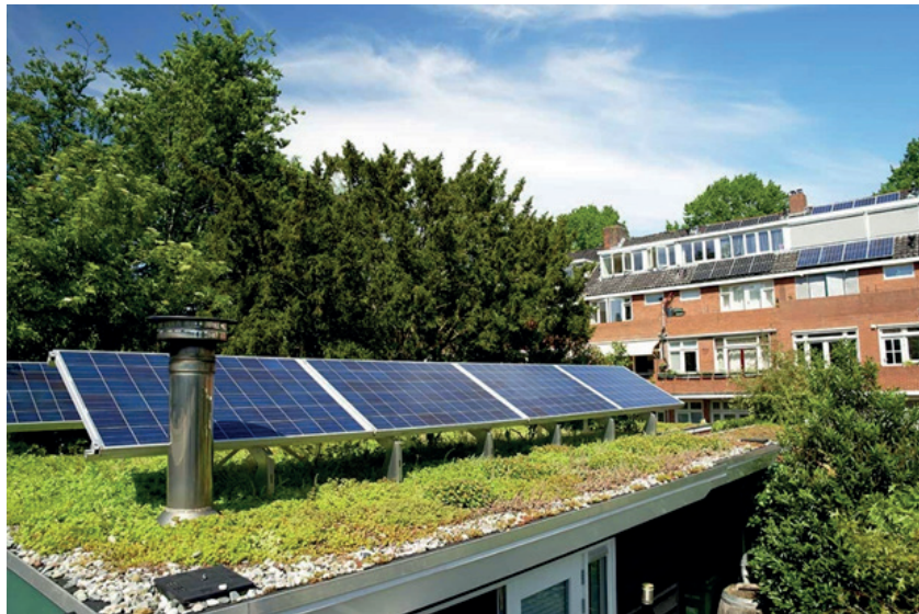
Example of a biosolar roof
