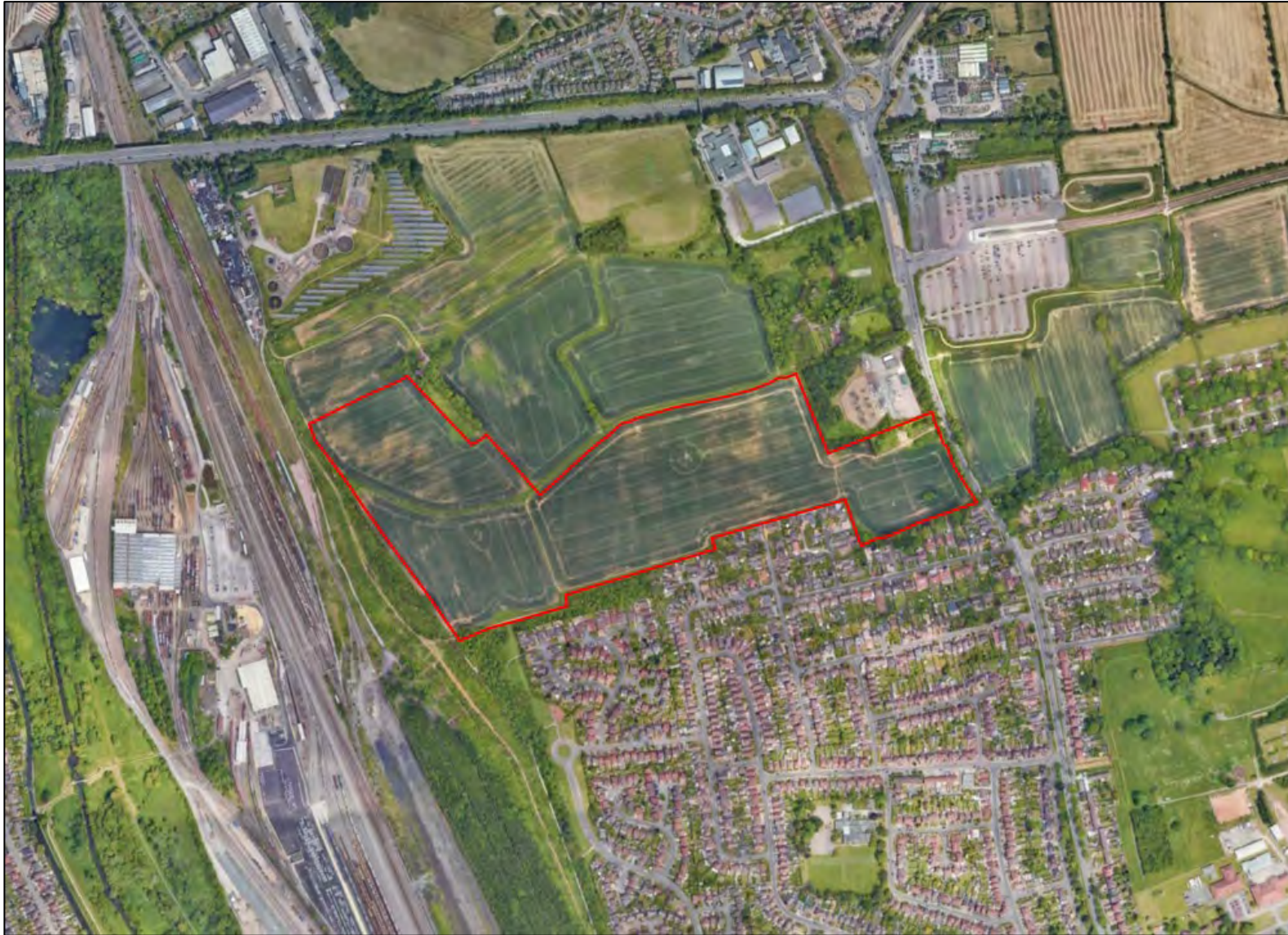
Plate 17: Extract from aerial photograph captured in 2022, with approximate site boundary edged in red.
