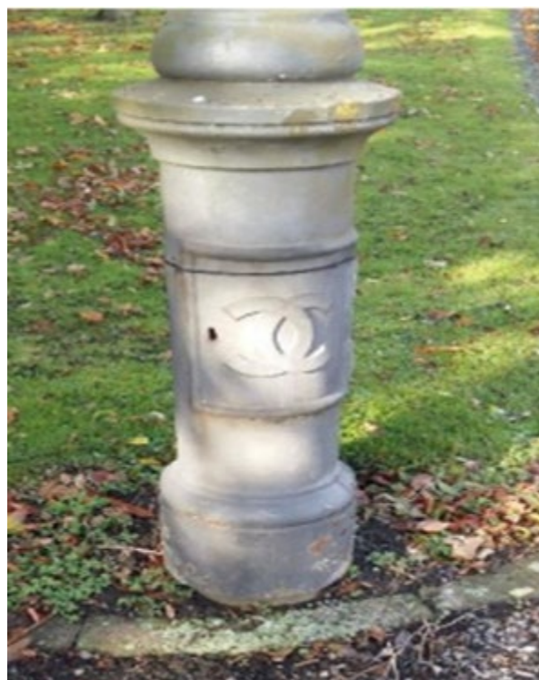
Example of the base of streetlamps in the Chetwynd Barracks site
