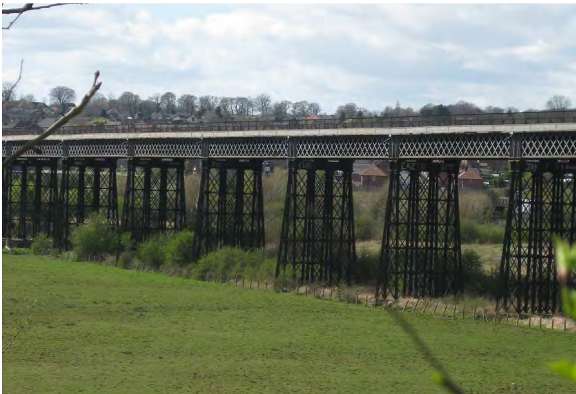
Bennerley Viaduct, Grade II* Listed Building.
