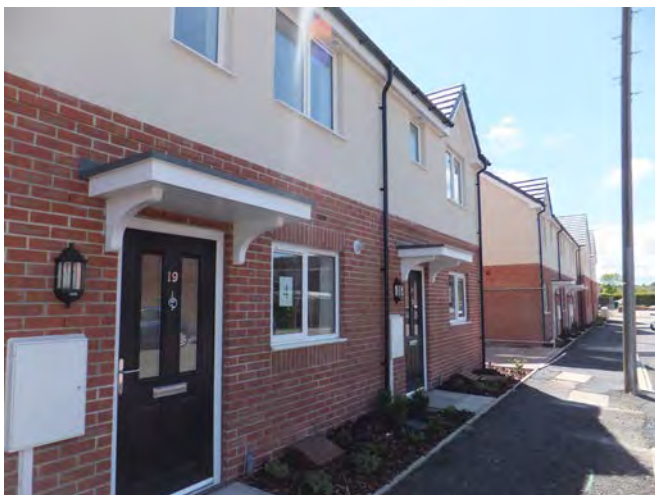
Peatfield Road, Stapleford, affordable housing
